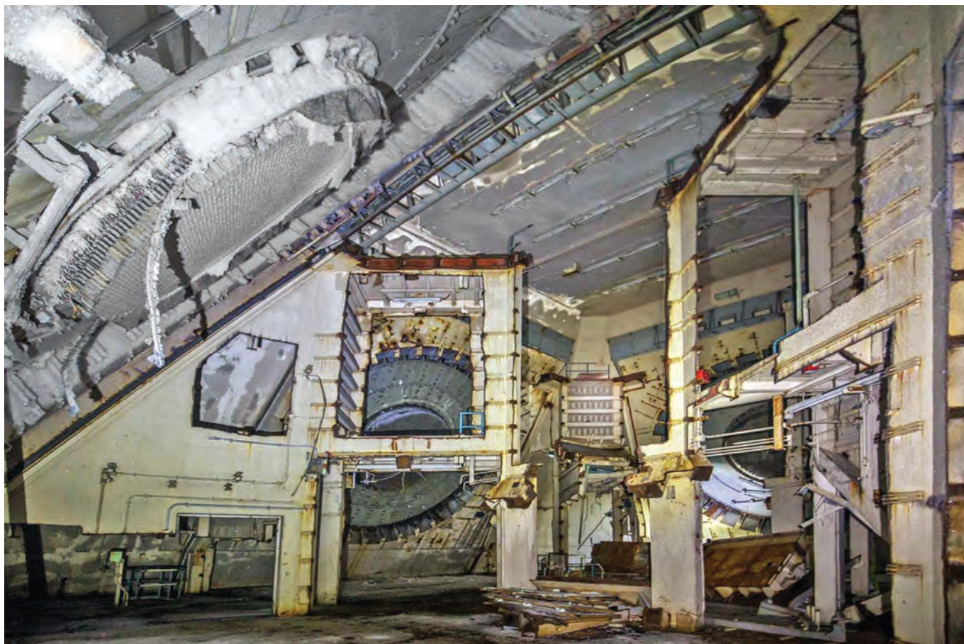
The Missile Site Control Building of the Missile Site Radar near the village of Nekoma, North Dakota. Interior view of level 4 showing three of the four antenna faces. Photo Chris Howells
